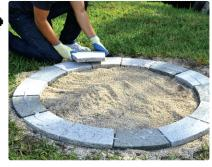
Once the first row is laid, apply a bead of high heat silicone to middle of stones and lay second row on top of first row (always rough side facing up), staggering joints as shown in picture above.
