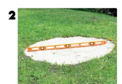
Put approx 2" of paver base into your circle - this MUST be tamped level before laying Encore Stones.
