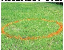
Select location for your fire pit, if using lawn/dirt location mark a 48" circle on surface and dig 2" down. Use level to ensure your base is even. If using existing patio surface, you can mark the circle with chalk (Not for use under covered patios or under trees). Now skip to step #3.
