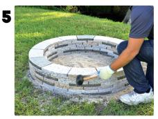
Repeat step #4 for rows 3-10, using the first 14 pieces you set aside for row #10 (Don't forget- install rough side up). Stop every 2 rows and use rubber mallet to tap any pieces that may have shifted before silicone fully cures.
